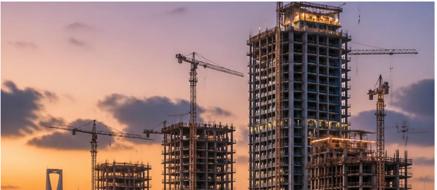
Hotel towers under construction in Saudi Arabia
